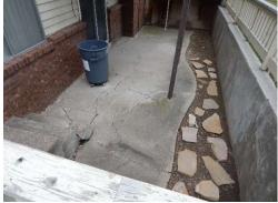
Concrete porches and patio areas on the property were generally in fair to poor shape as of the date of our review. The replacement of the concrete will be a major repair and currently the expected useful life would be typical for the conditions of this area. Recommend a sytematic process of replacement every 3 years until the property has been restored to its original state of repair. This estimate may need to be revised as wear and tear is monitored in the coming years.
