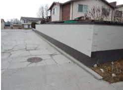
The masonry wall was constructed at the time the property was completed. It is a painted cinder block wall. We would expect this wall to last as long as the property is in existence. No reserves needed for the wall.
