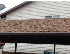
Roof is 30 yr architectural shingles which show serious signs of wear. Both of the carports by the buildings that were involved in the fire in 2012 were affected by the heat and are in need of replacement. Recommend full replacement immediately along with gutters and downspouts to take advantage of economies and ensure proper long term functionality.
