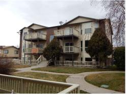
Concrete sidewalks on the property were generally in fair shape as of the date of our review. The replacement of the concrete will be a major repair and currently the expected useful life would be typical for the conditions of this area. Recommend a systematic process of replacement every 3 years until the property has been restored to its original state of repair.
