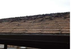
Roof is 30 yr architectural shingles which show serious signs of wear. Both of the carports by the buildings that were involved in the fire in 2012 were affected by the heat and are in need of
