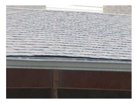
The roof was inaccessible at the date of our review. Recommend full replacement after 27 years along with gutters and downspouts to take advantage of economies and ensure proper long term functionality.
