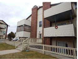
The decks were in reasonable condition as of the date of our review. The decks are made of wood for the deck and railings, the joists are wood. Recommend a periodic replacement of the decks to maintain the asthetic value of the property.
